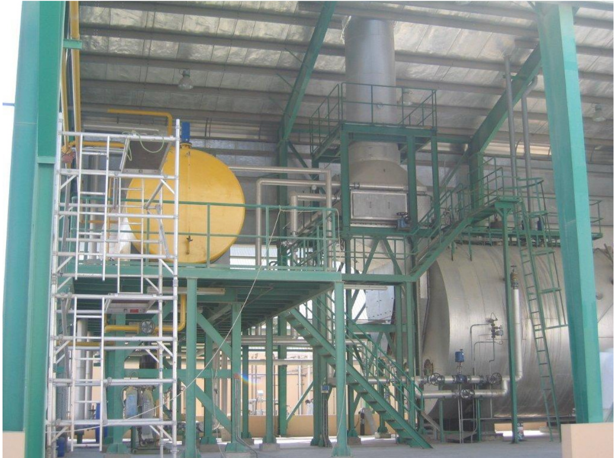
Steam Boiler Plant
